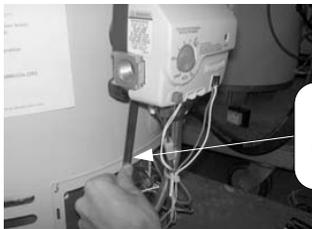
With service tool inserted, pivot tool back towards heater as far as possible. Lift straight up on control, control will move 1/8". Remove tool and continue to lift straight up on control to remove from Thermal Well.
